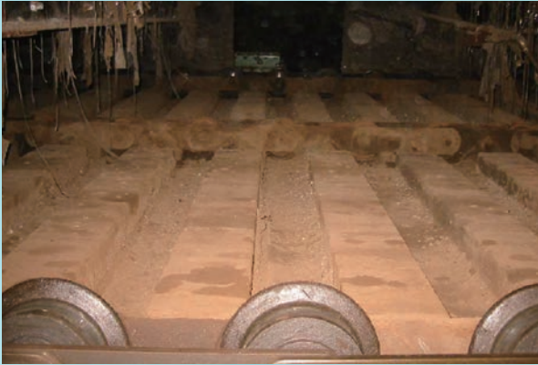
Bulky Trash Feed Conveyor
