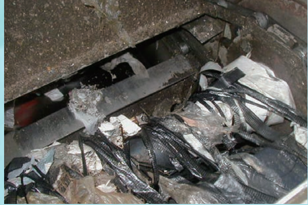
Crushed Matter Conveyor
